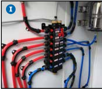
The Water Distribution Manifold is pre-set at the factory. DO NOT ADJUST!
