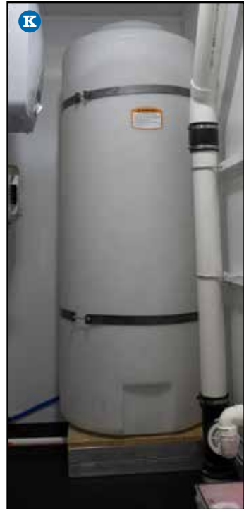
On-Board Fresh Water Tank —105 gallons
